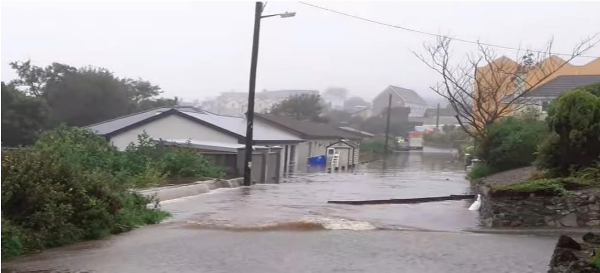
Clifden Flood Relief Scheme – Flood Waters, Clifden September 2020
