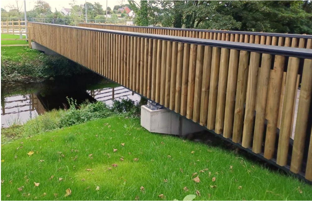
Athenry Footbridge completed in 2022
