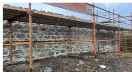
Fig. 2 Site Setup (GAA side of wall)
