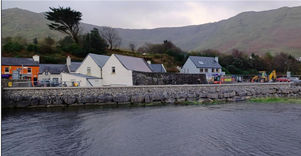
Coastal Defence Works completed at Leenaun Village 2022
