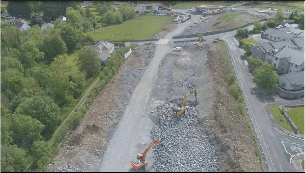
Rock Breaking at Cut 02 Adjacent Knockferry Road
