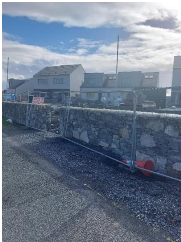
Under Construction photo from Garrai Ghuaire October 2022
