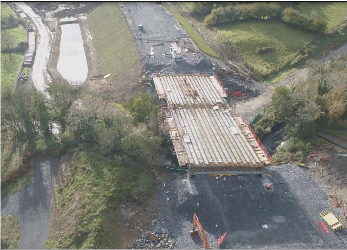
Ariel View of ST07 Lough Kip River Bridge
