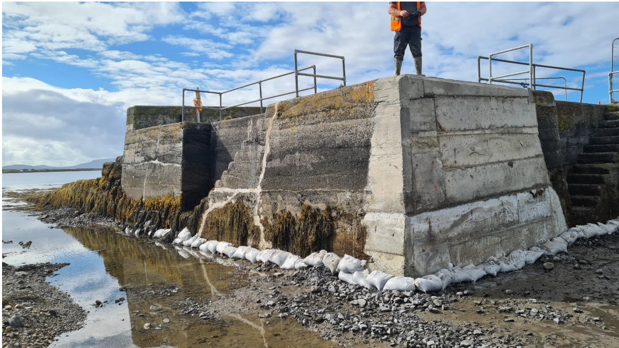
Completed Works at Blackweir Pier - BALAMI Funded Project
