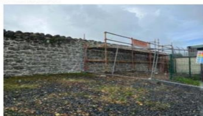
Fig. 1 Site Setup (GAA side of wall)
