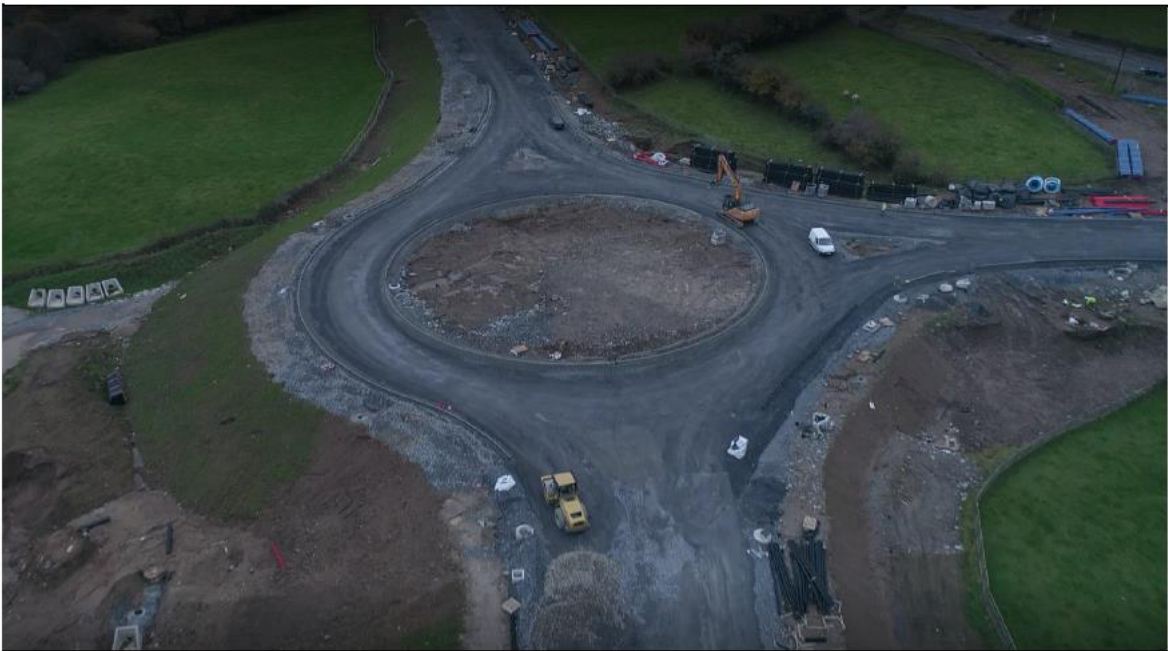
Kerbing & Utility Ducting Installation at Eastern Roundabout at Clydagh
