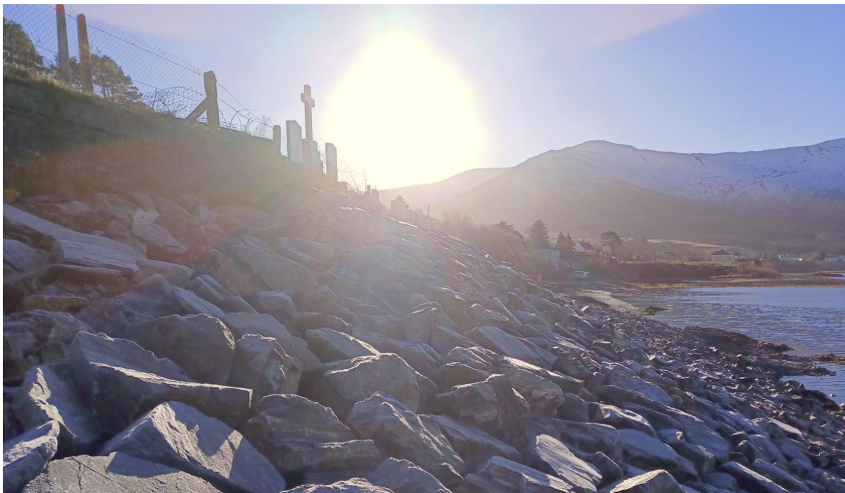
Coastal Defence Works completed at Leenaun Graveyard 2022
