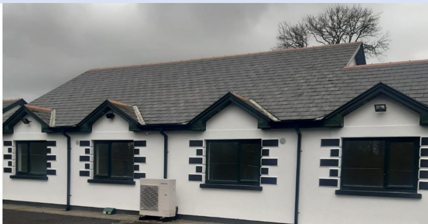
Major refurbishment at Energy Retrofit to Traveller Specific House
