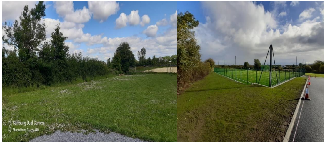
Image: Lurga National School - Supply & installation of 45m x 30m Astro pitch for community use adjacent to Lurga NS.
